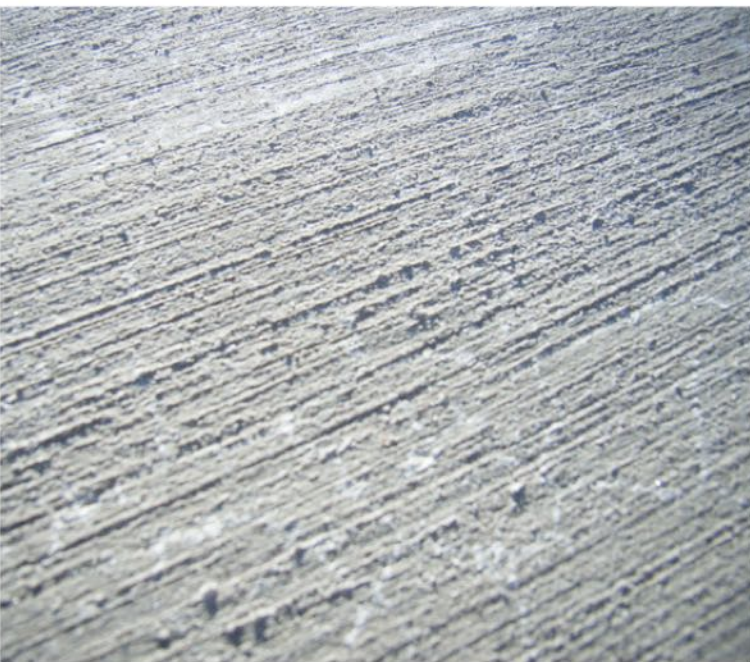
Broom Finish Concrete
