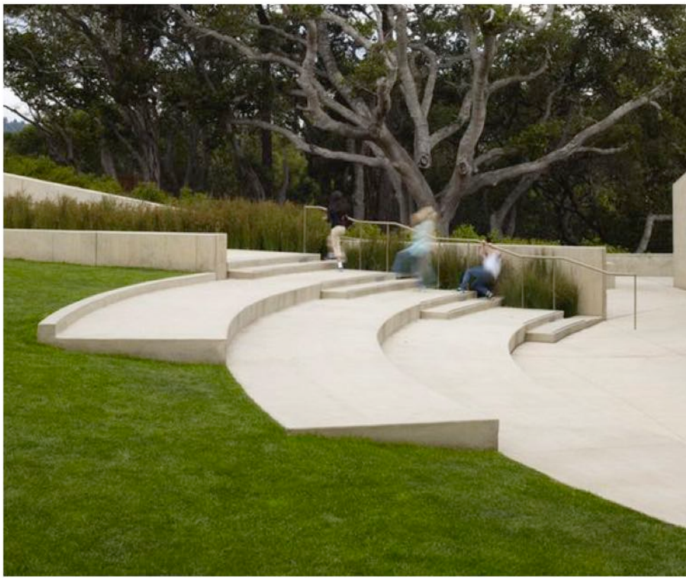
Concrete Retaining Wall & Staircase
